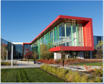
9 The Linx Office Complex
