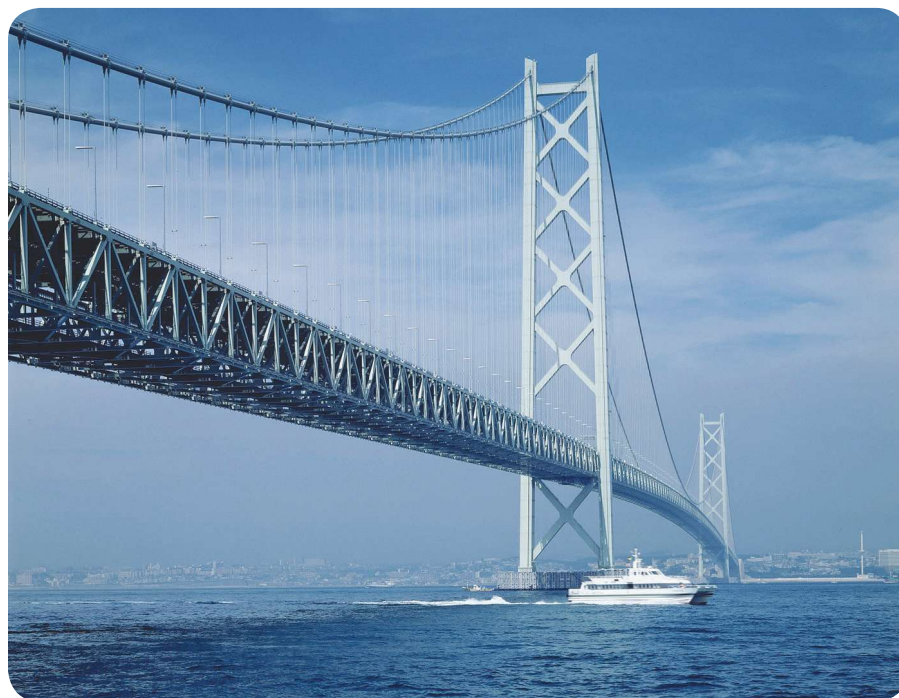
FIGURE 2 Shown is the Akashi Strait Bridge in Kobe, Japan. Bridges like this are susceptible to corrosion from UV exposure, wind, and extreme and fluctuating temperatures. FEVE resins provide the needed protection.
