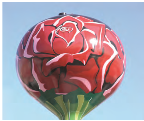
Fig. 2 Fluoroethylene vinyl ether-based topcoat used on the Rosemont Water Tower near the Chicago O'Hare International Airport. Courtesy of Tnemec Company, Inc.
