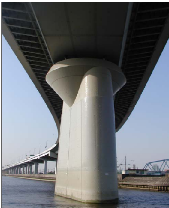
New Steel Encasement: Coated 2007
