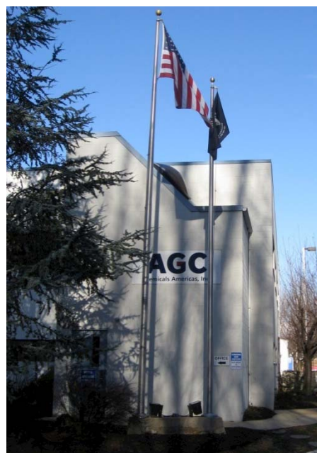
Thorndale Manufacturing 255 South Bailey Road Downingtown, PA 19335 Phone: 610.380.6200
