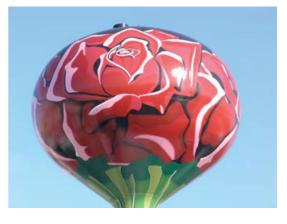
by sketching it in pencil directly onto the tower using photographs as a reference. He spent several weeks applying the finish coat, using 9-inch rollers to apply the finish coat wherever there were solid colors, like on the riser, and used 4-inch rollers and dozens of 2.5-inch sash brushes for the detailed work.
