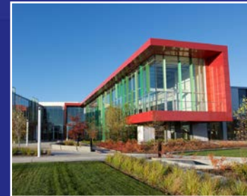
9 The Linx Office Complex
